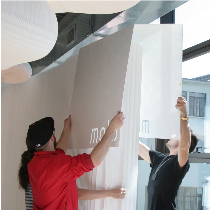
laser-cut textile saddle-sign being installed over softwall.
